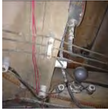
Knob and Tube Wiring
