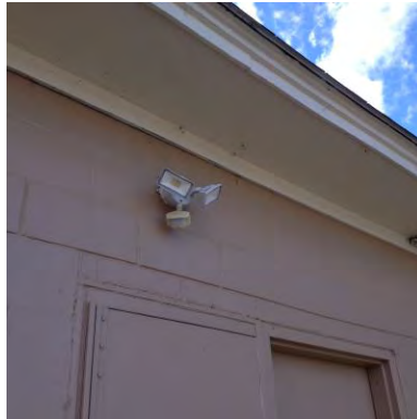
LED Mini-Floods with PIR Sensor
